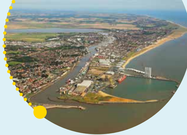
Above – Aerial view of Great Yarmouth port ( Credit: Mike Page)
